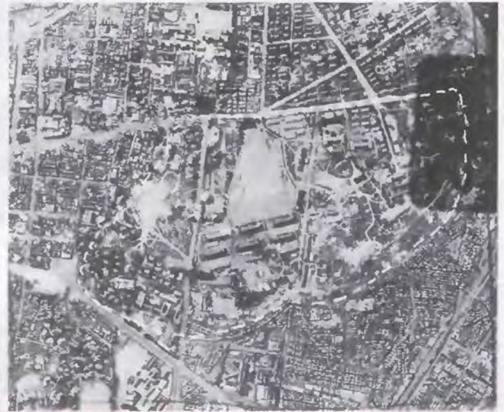
Bombardiers of the Far East Air Forces Bomber Command are proud of the precise plastering they gave three Communist Military Barracks and Training Centers in and near Pyongyang on September 20, 1950. The barracks, where Red reinforcements were being assembled, were surrounded by civilian homes. This required that these targets be hit without damage to surrounding areas.
