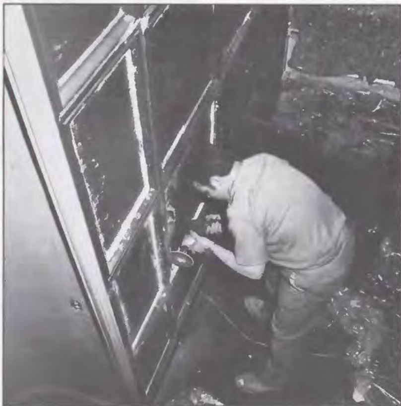
Publications Department's Ron Pine removes old paint from lobby walls.
